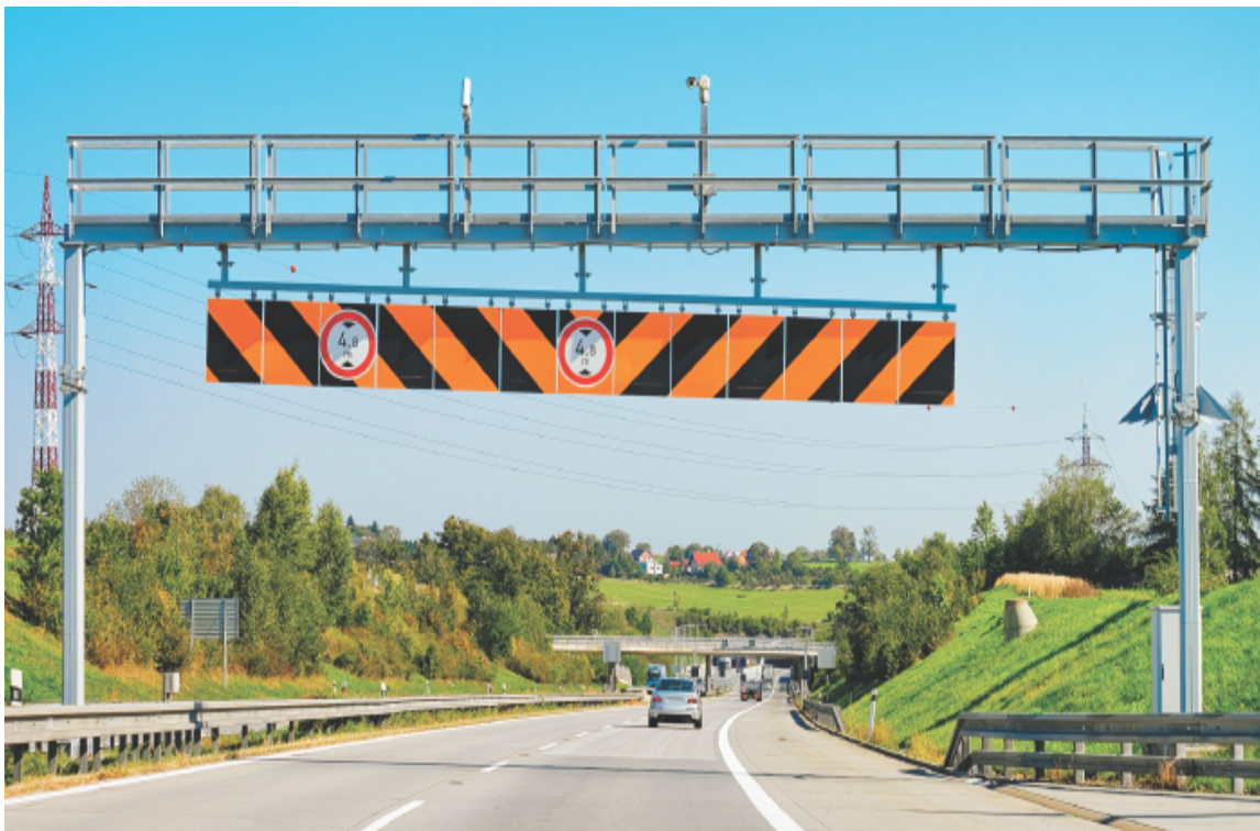
Figure 8.4 A height restriction barrier. Light-weight bars hang from chains. A truck too tall for what's up ahead will first hit these bars, with much noise but little damage.
